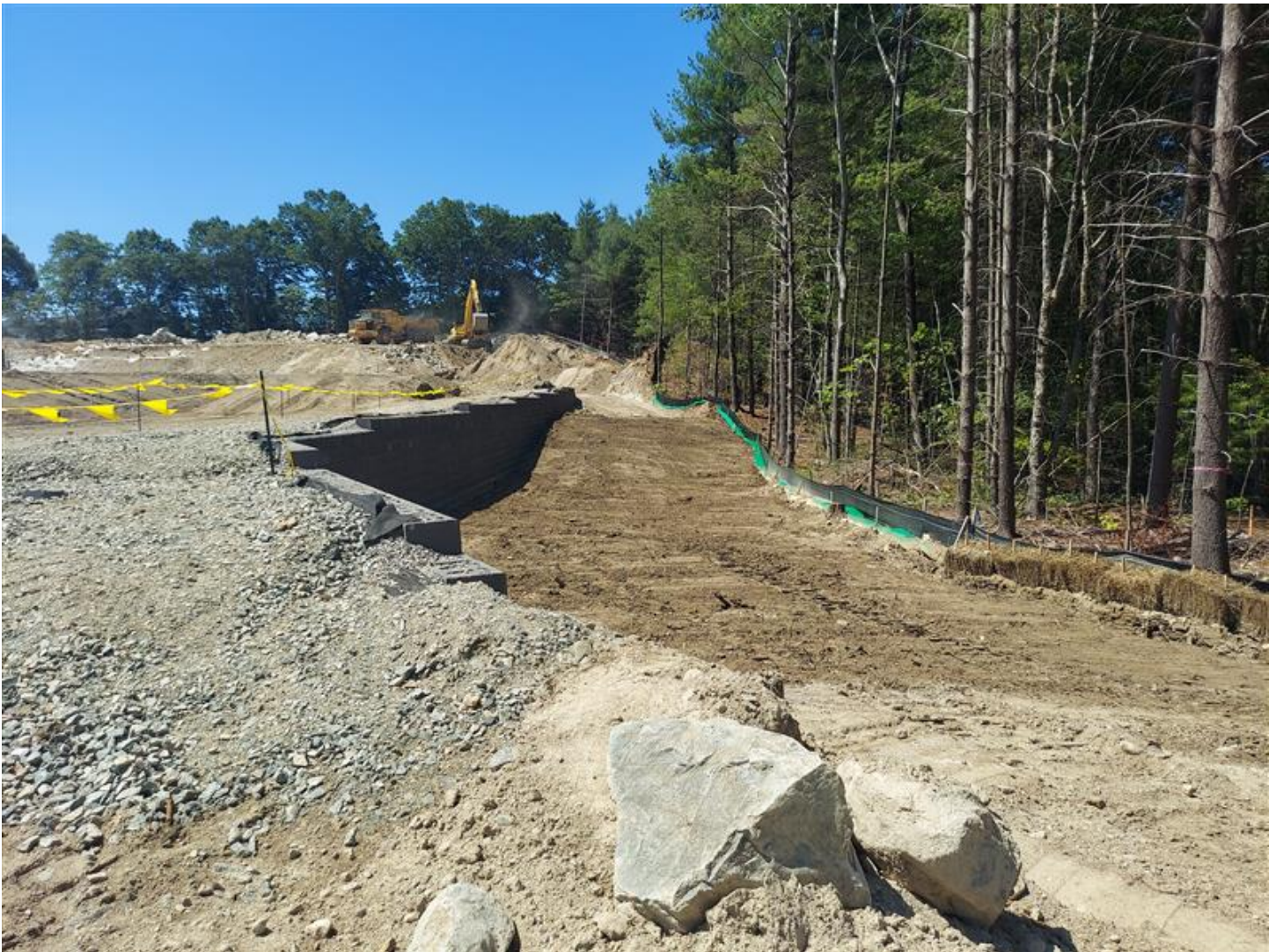
Photo 2: In progress view of retaining wall installation at a development site
