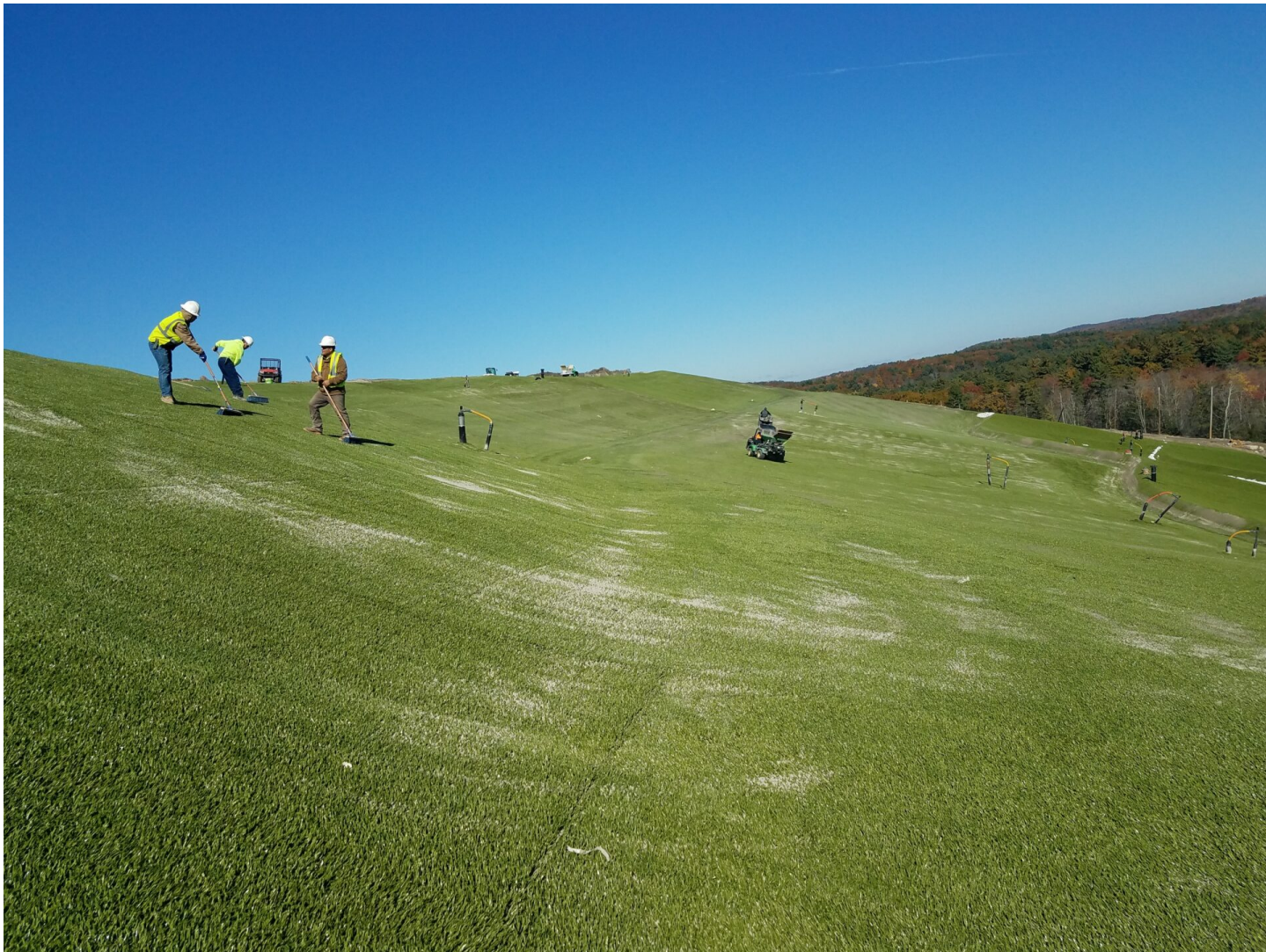
Image 1: Installation of ClosureTurf® system at the Southbridge Recycling & Disposal Park in Southbridge, MA.
