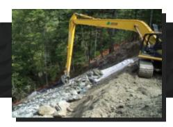
Sanborn Head provided geotechnical engineering services for emergency repairs to Bethel Mountain Road following extensive damage sustained during a heavy rainfall event in the spring of 2019. Damage included washed out culverts, soil slope failures impacting the edge of roadway, extensive pavement damage, and loss of roadway guard rail.
