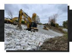
Sanborn Head provided engineering, design, and construction phase services to the Town of West Rutland, Vermont to repair a soil slope that experienced excessive movement after a significant rainfall event and subsequently damaged an adjacent roadway.
