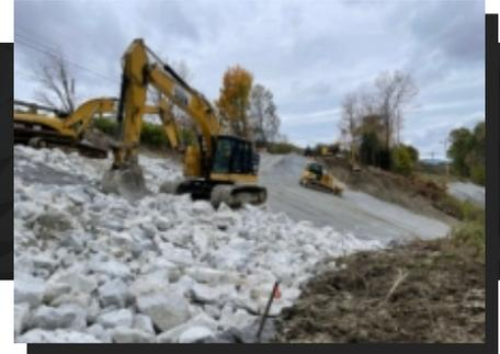
Sanborn Head provided engineering, design, and construction phase services to the Town of West Rutland, Vermont to repair a soil slope that experienced excessive movement after a significant rainfall event and subsequently damaged an adjacent roadway.
