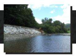
Sanborn Head provided engineering and construction phase services to the Town of Bethel, Vermont to repair a soil slope adjacent to Peavine Boulevard. The slope sustained damage during a flooding event caused by heavy rains.
