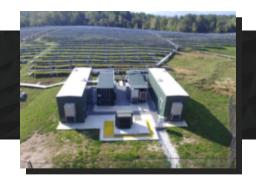
Sanborn Head provided engineering and geotechnical services for the design, permitting, and construction of a 2.3 megawatt (MW) solar project for Green Mountain Power Corporation on a closed landfill in Rutland, Vermont. The project included the installation of battery storage on the closed landfill and was configured as a microgrid.
