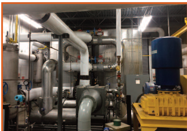
Figure 2. Regenerative Siloxane Removal System Installed at an LFGTE Facility.
