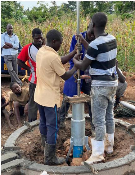
*Pump being lowered into a newly installed water supply well. (Credit: Habert Ongom, Engineers Without Borders Uganda Country Office)*
