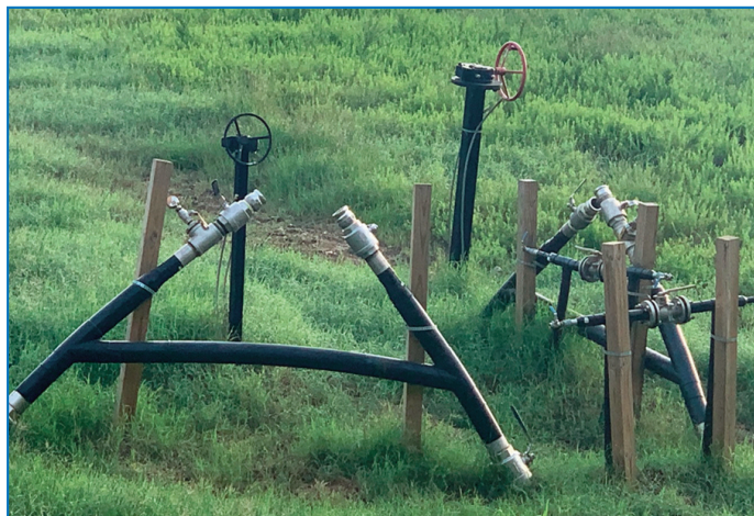
Figure 2. Example of a pipeline high point that needs an air release valve to eliminate air locking.
