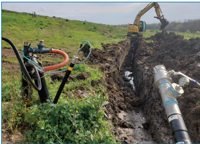
Figure 1. Excavation in the landfill for leachate force main installation.
