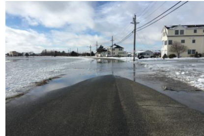
High Tide Flooding Impacts Require Improvements to Tidal Drainage Systems
