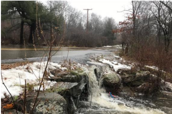
Undersized Culvert Overtopped Due to Heavy Rain
